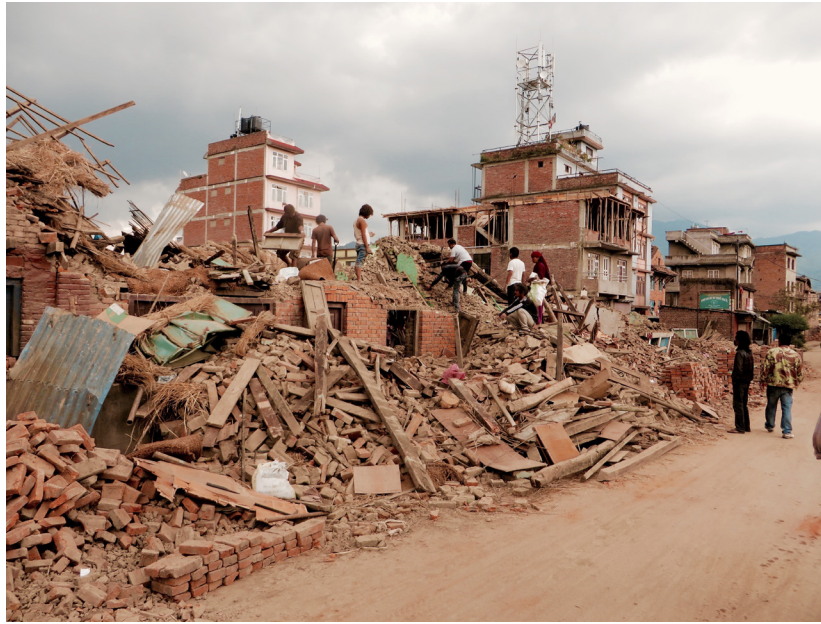
Aftermath of Nepal Earthquake – Photo by simcsea via Flickr.
