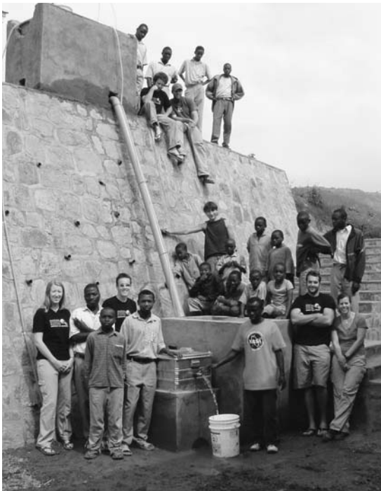
FIGURE 10. The completed BYOW Treatment Systems installed at the Muramba Clinic in June 2006.
