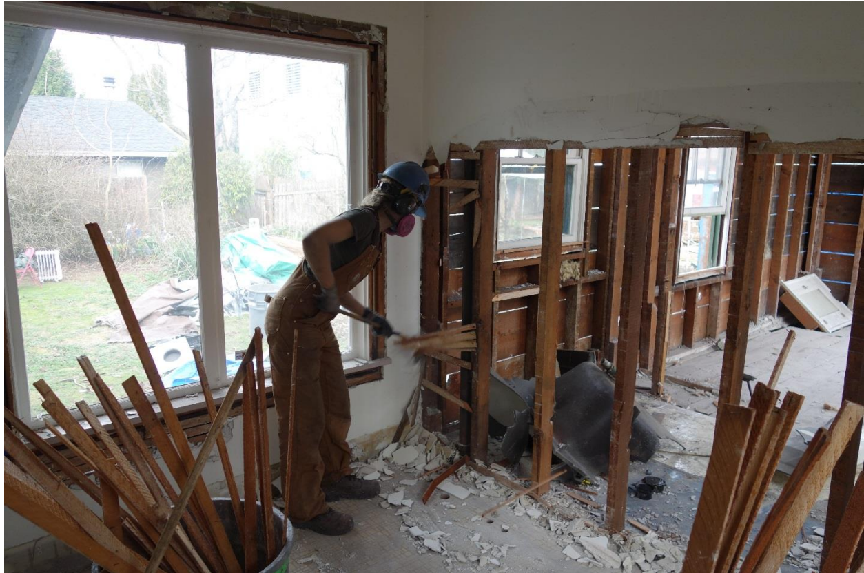
Photo: Lovett Deconstruction
