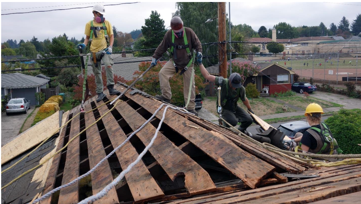
Photo: Lovett Deconstruction
