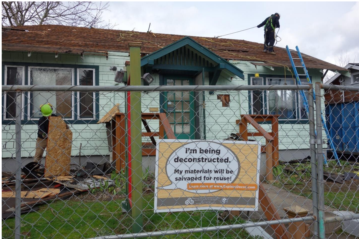
Photo: Lovett Deconstruction
