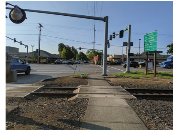
Pedestrian rail crossing at the intersection of Highway 30 and Gable Road
