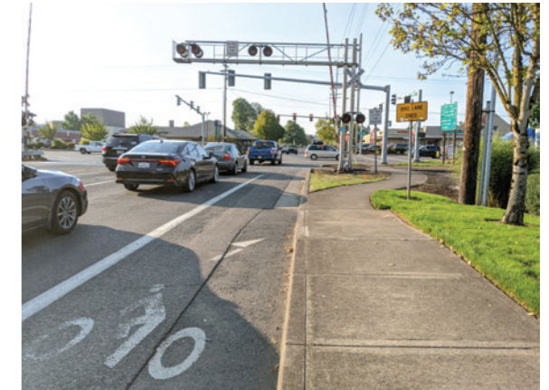
Unprotected bike path at the intersection of Highway 30 and Gable Road
