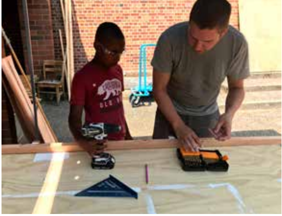
Constructing walls for KSMoCA International Art Fair led by Spencer Byrne-Seres with MLK Jr. School Students, KSMoCA, Portland, OR, 2017
