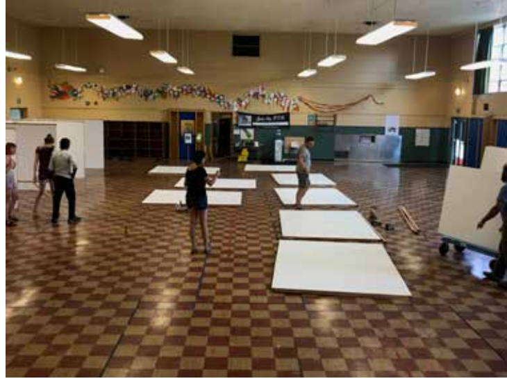
Installing walls for KSMoCA International Art Fair led by Spencer Byrne-Seres with MLK Jr. School Students and volunteers, KSMoCA, Portland, OR, 2017
