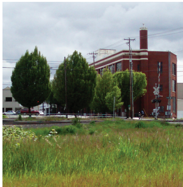
Ford building and grassy lot adjacent Union Pacific Railway
