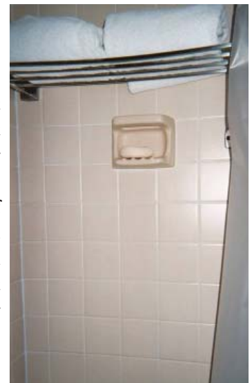
Elevated soap dish within shower area.
