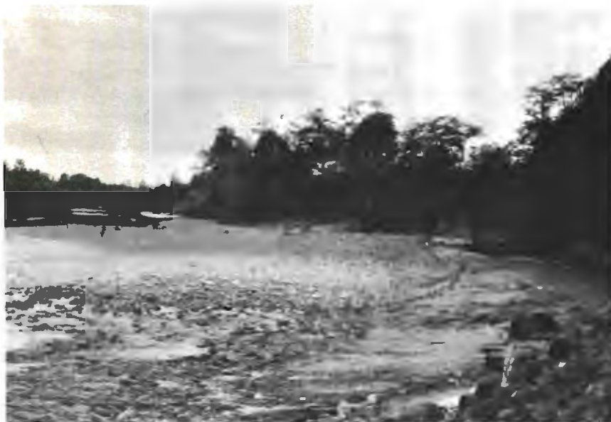
Fig. 13-A Channelization along the outside of a meander on the Kilchis River. The rock protects the easily eroded silt banks, preserving farmland and reducing the amount of deposition in Tillamook Bay.
