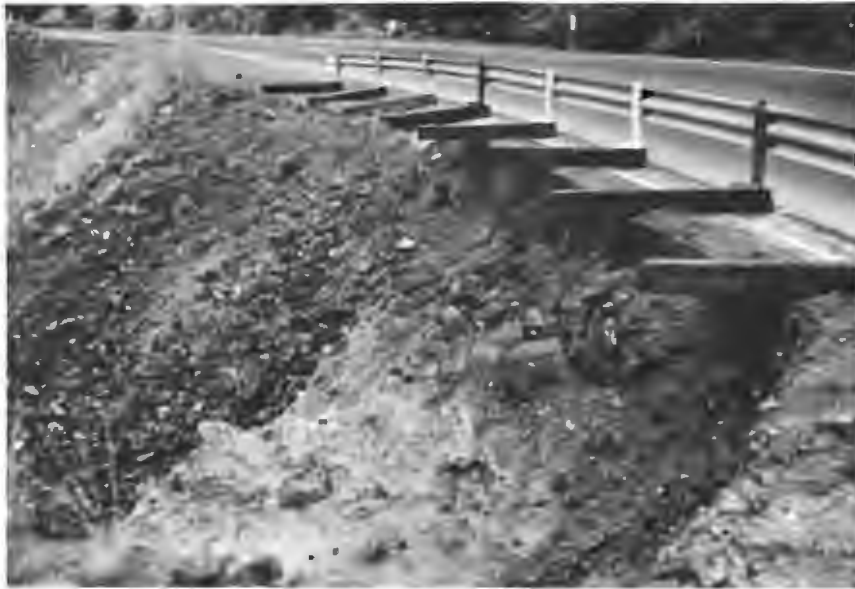
Fig. 4-A The combination of heavy rain, steep slopes, and unstable materials create continuing slide problems as can be seen on this section of highway a short distance east of the summit. (Mile 37.3)
