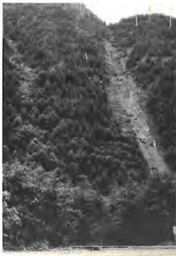
Fig. 8-B The fresh scar on the steep hillside is an area of active and rapid downslope movement. To the left is an older slide partially healed by vegetation. (Mile 45.3)
