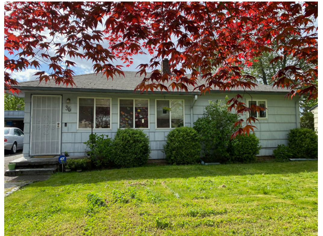
Top: The front facade of the Portland Conservatory, 2020.
