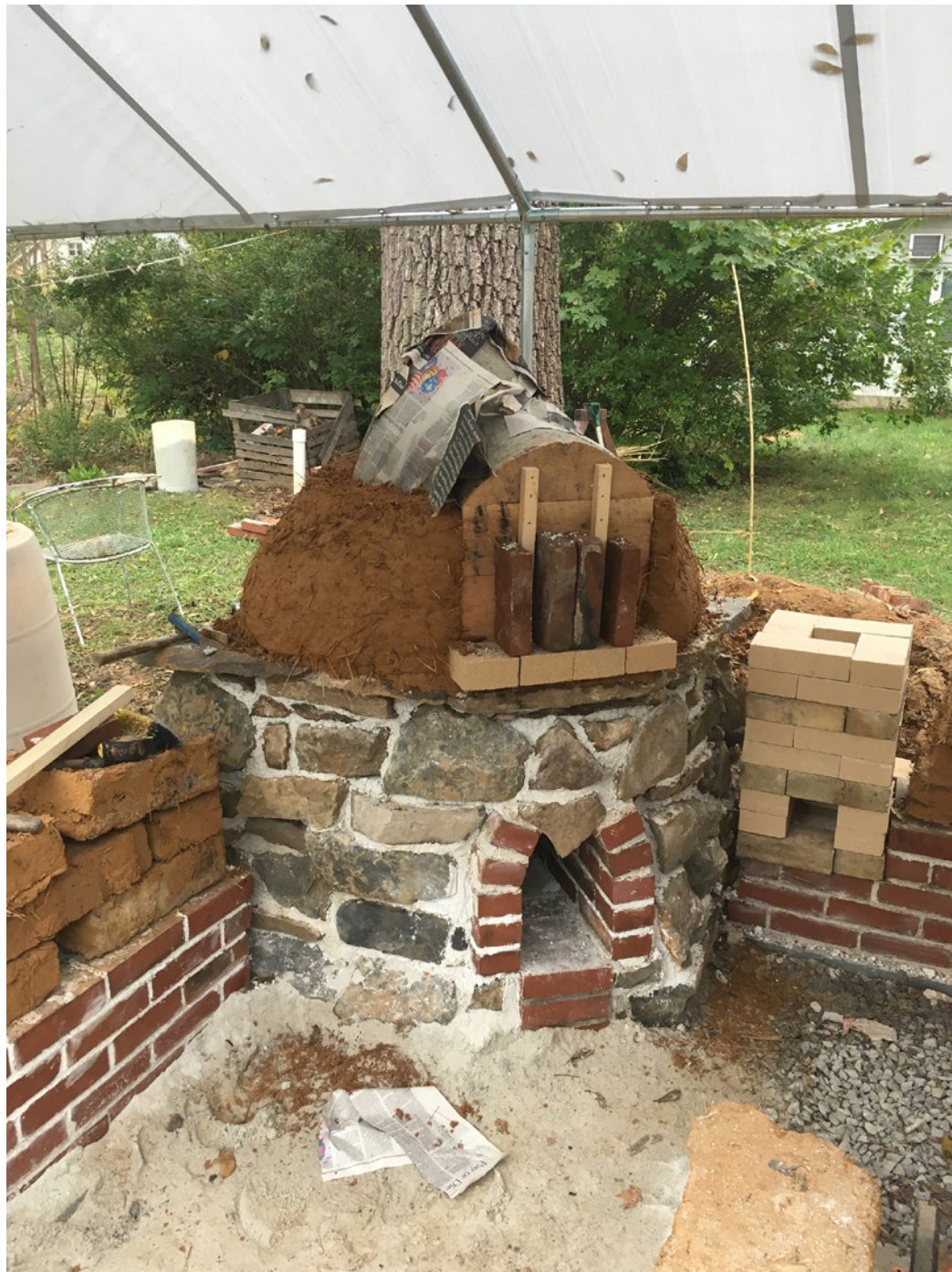
Top: Process image of a wood-fired cob oven project: made from earth, stone, sand, straw, and bricks. Submitted to the archive by Jeff.
