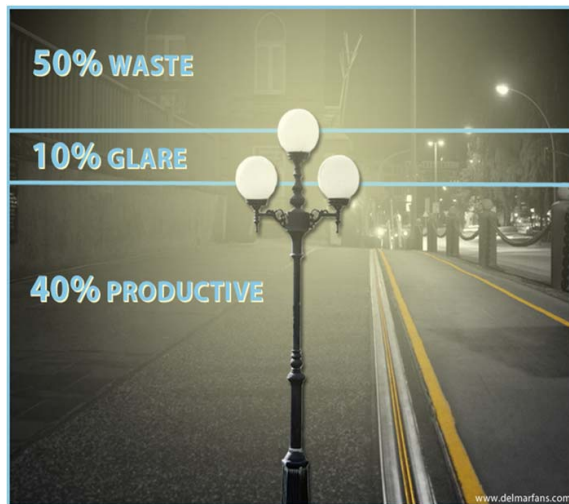
Figure 1: The use of an ordinary street light produces more waste than effective lighting
