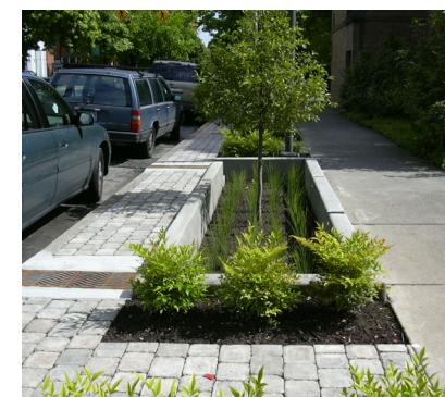
Example: Sidewalk swales add greenery while buffering traffic and provide sustainable stormwater management
