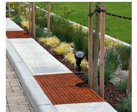
Example: Sidewalk swales add greenery while buffering traffic and provide sustainable stormwater management
