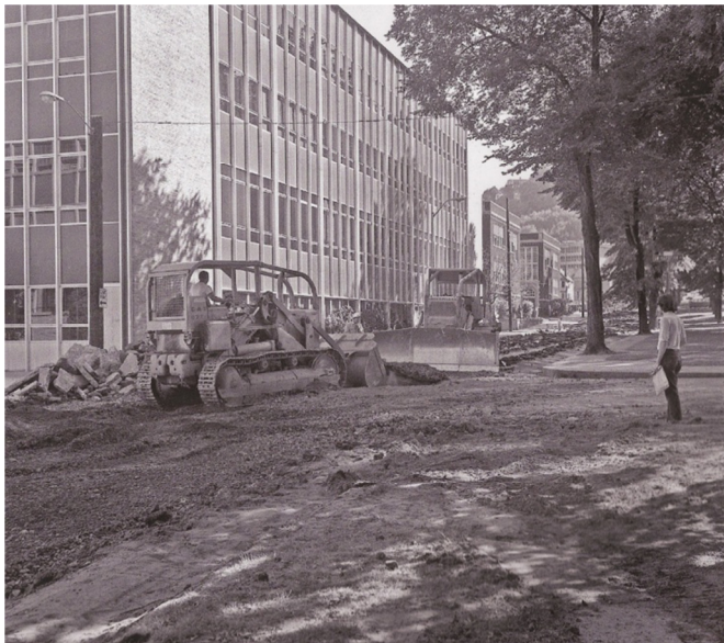
Before: Bulldozers remove pavement in the Park Blocks by College Center (now Smith Memorial Student Union) in 1972.
