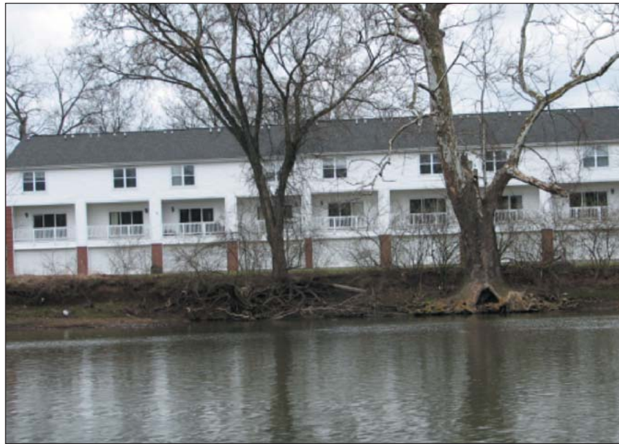
Figure 7. One possible future development pattern for areas at risk for flooding, with non-essential activities (such as garages and parking) on the ground floor.
