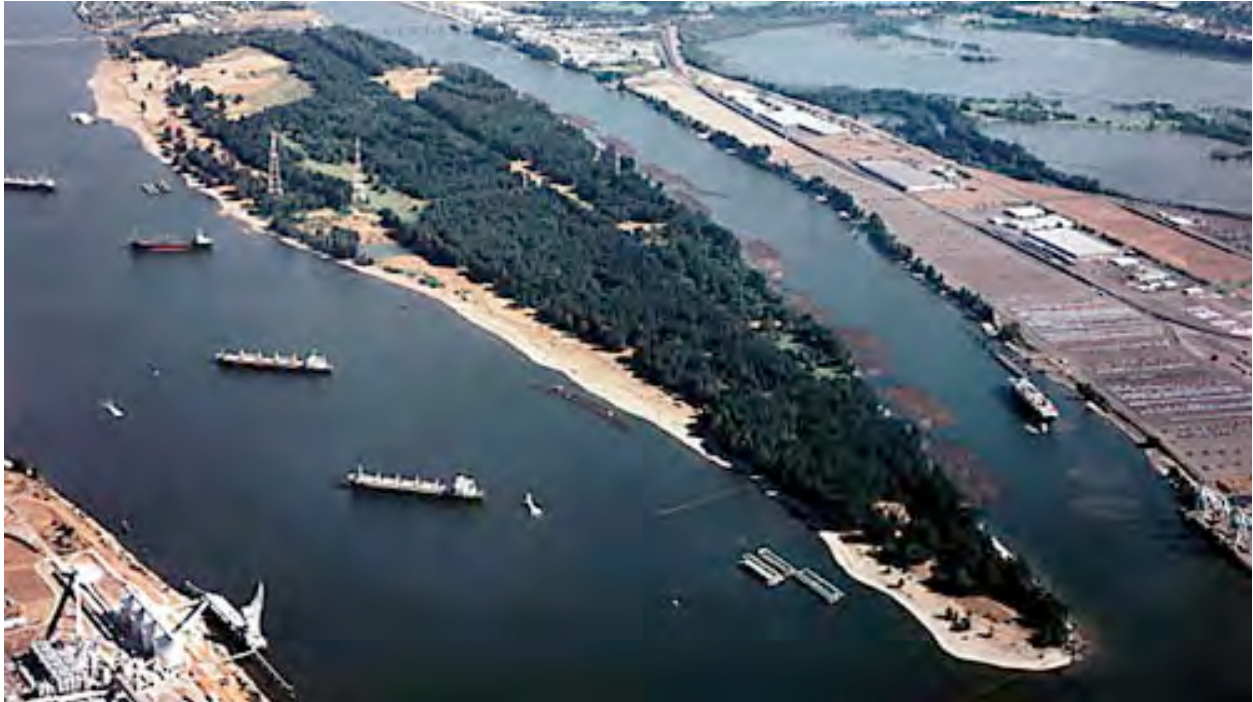
Before Port Development
