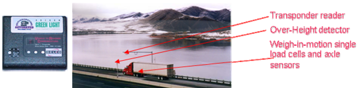
Figure 3.1: A Green Light RFID Transponder and Station Pre-clearance Arrangement
