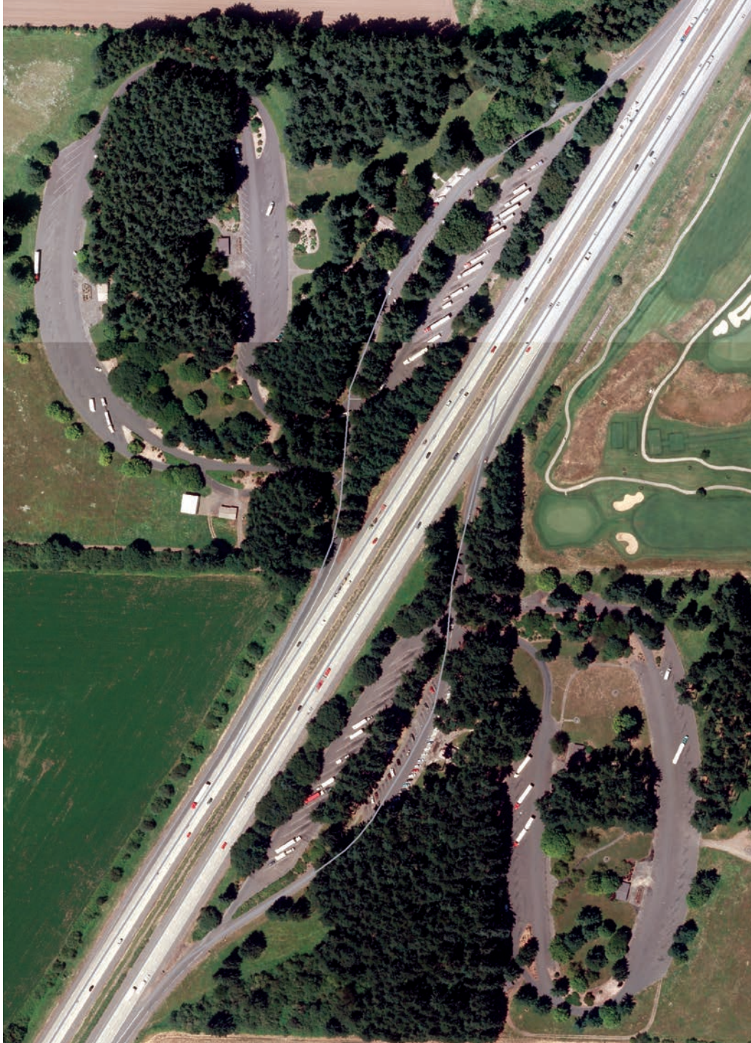
The Baldock north and south bound rest stops off of I-5 near Wilsonville, Oregon.
