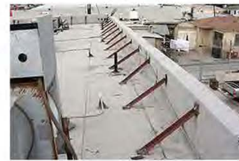
Roof Parapet Bracing
