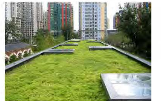
Green Roof w/ Skylights
