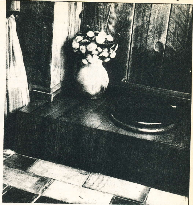
Farallones' most recent composting privy, with seat and platform built for squatting or sitting.
