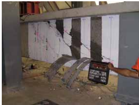
Figure 5.19: Failure photograph of Specimen IT12FTCK
