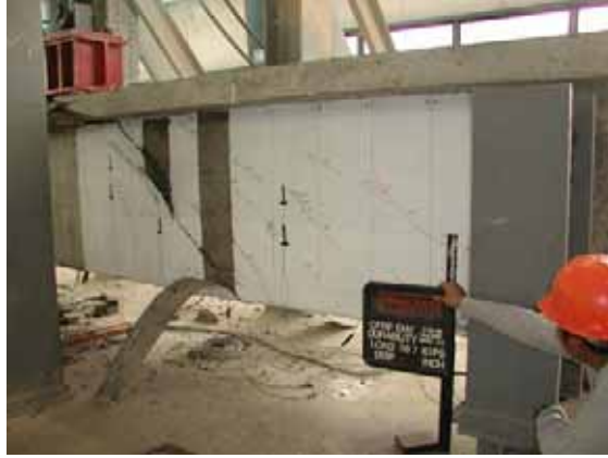
Figure 5.18: Failure photograph of Specimen T18FT
