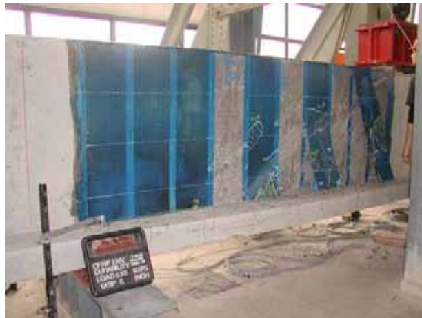
Figure 5.11: Failure photograph of Specimen IT12Control
