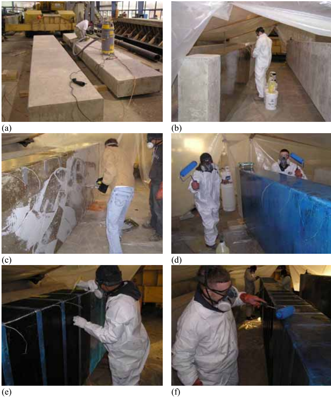
Figure B-4.3: CFRP application process
