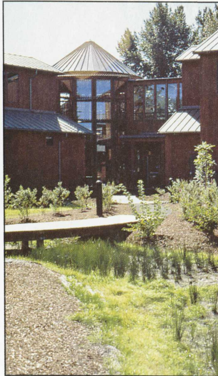
USA's innovative design features demonstration bioswales (foreground) which filter stormwater runoff from the adjacent parking lot and rooftops.
