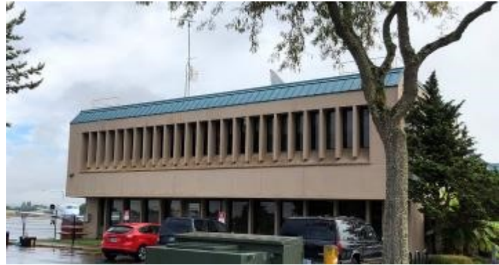
Airport terminal building
