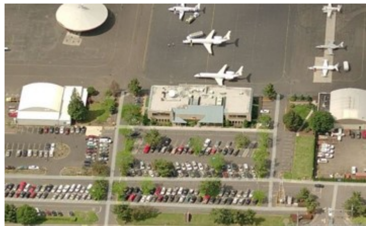
Airport terminal building with apron
