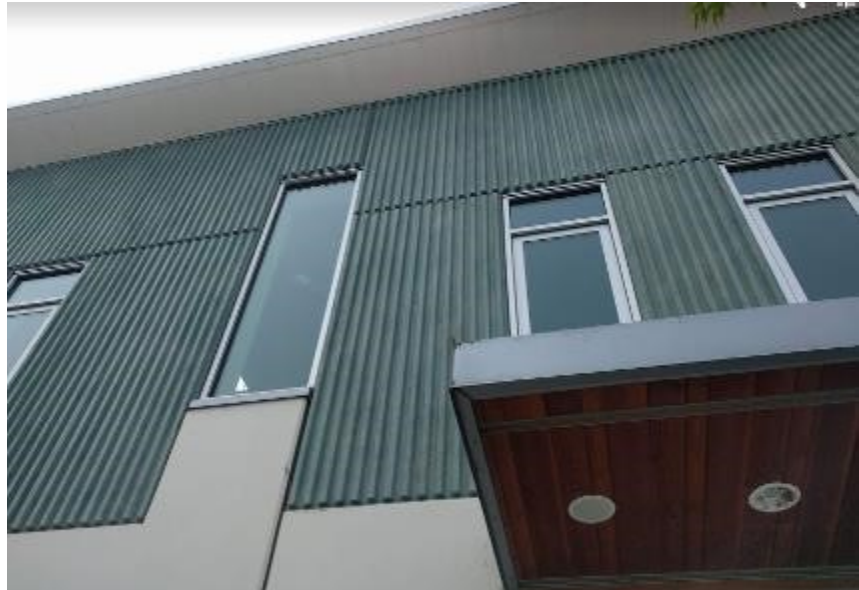
Example of Cargo Hold's façade material
