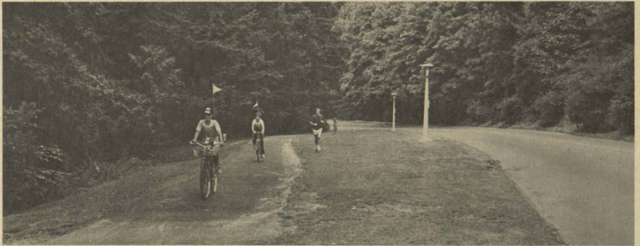
Bicyclers and a jogger are separated from traffic flow on the Terwilliger Blvd. Bikeway (Class I). The facility is 3.9 miles long and cost approximately $370,000 in 1973.
