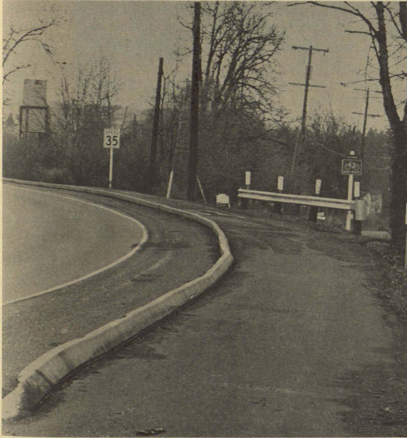
A Class II Bikelane with extruded curbing, located on State Highway 43 between West Linn and Lake Oswego. Facility permits two-way bicycle traffic on one side of the highway.
