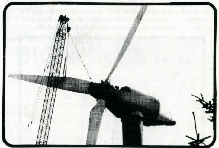
November 17, 1977: bolting on the last 88½ ft. blade, 2½ years after May 29, 1975, ground-breaking (note size of workers atop rotor hub and in open nacelle).
