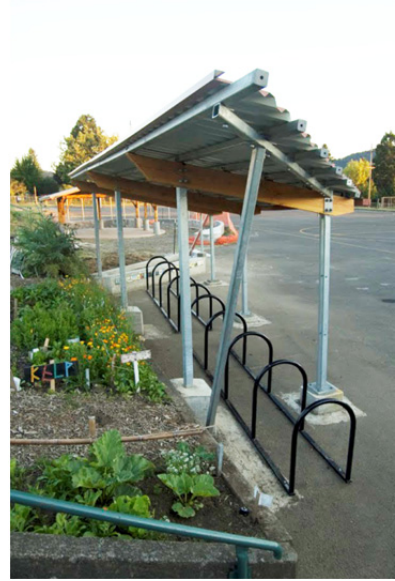
Steel purlins and roof installed.
