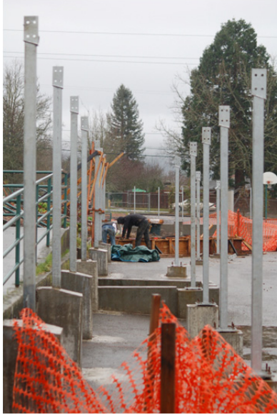
Forms stripped and columns aligned.
