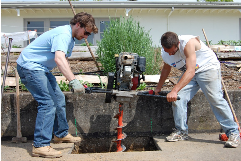
Following concrete sawing, Nick Venezia and Henry Malmberg excavate for footings.
