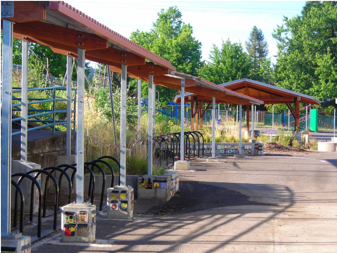
Photo of Camas Ridge Pedal, facing south toward the outdoor classroom. Hidden from view here, steps to the Learning Garden are located between two separate bike-shelter elements.
