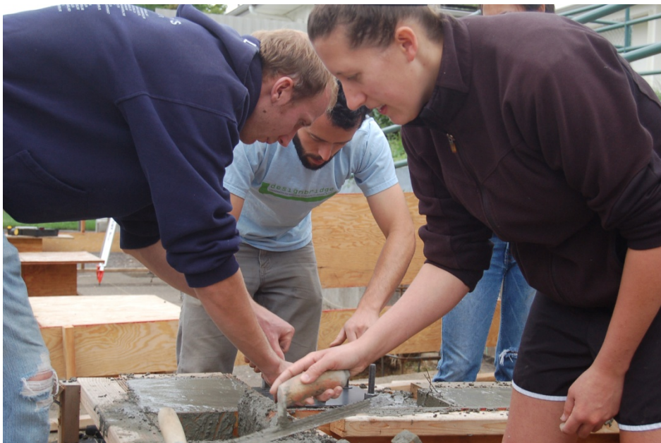
Troweling concrete to top of formwork at planter beds.
