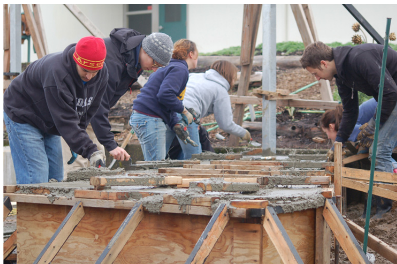
Column bracing assures that they will remain in proper place during the concrete pour. During the pour, students focus on sloping the tops of column bases for drainage and placing connectors for the front row of columns.
