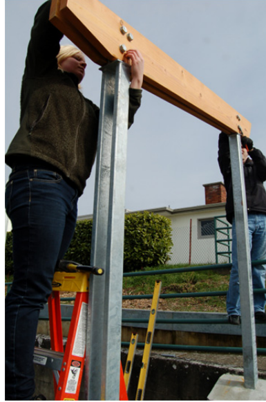
Fastening beams to columns.
