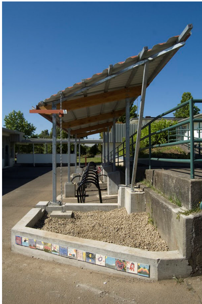
Looking north toward Structure One from the planter bed and stairs.
