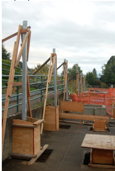
Column bracing assures that they will remain in proper place during the concrete pour. During the pour, students focus on sloping the tops of column bases for drainage and placing connectors for the front row of columns.
