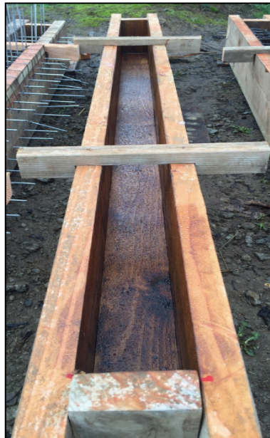
Figure 10: Plain concrete mold
