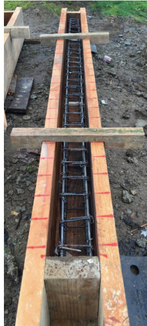
Figure 11: Reinforced concrete beam mold
