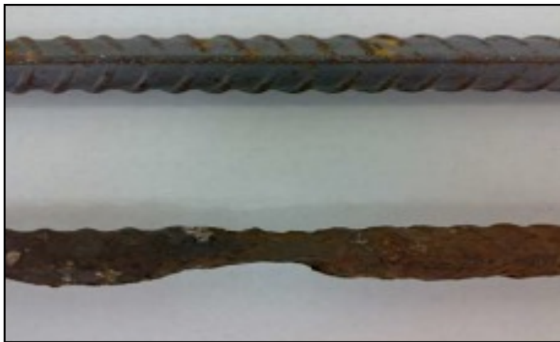
Figure 5: Corroded steel bar in comparison with noncorroded steel bar [14]
