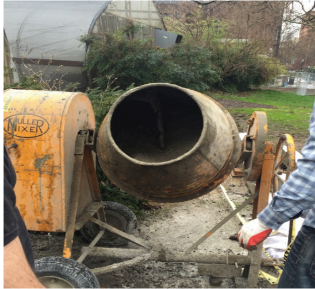
Figure 13: Mixing concrete on sit
