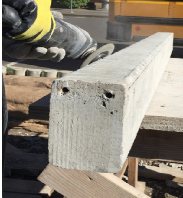
Figure 18: Beam surface and corner preparation
