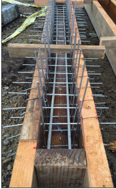
Figure 9: Deteriorated beam mold
