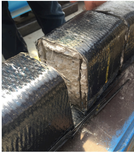
Figure 35: Beam #5 shear failure
