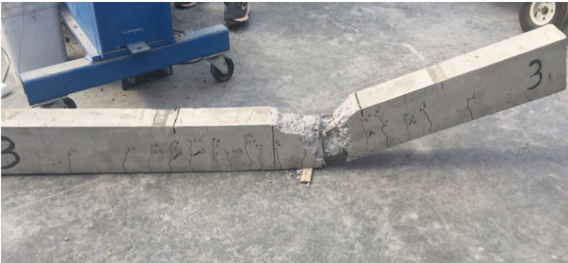
Figure 31: Yield of steel reinforcement in beam #3
