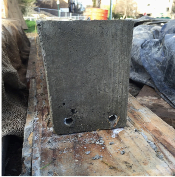
Figure 16: Voids representing deteriorated flexural reinforcement
