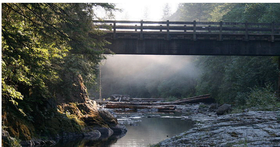
Bridge over Washougal River, WA
