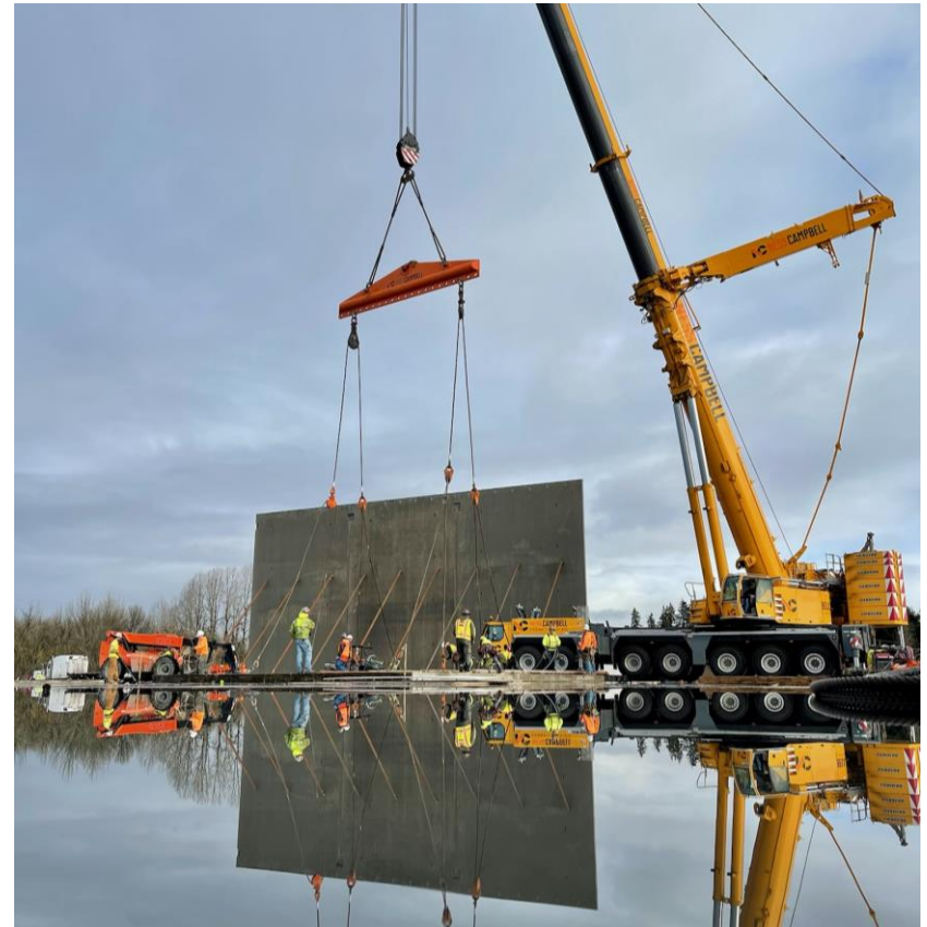
Panels are set into place with a crane.
