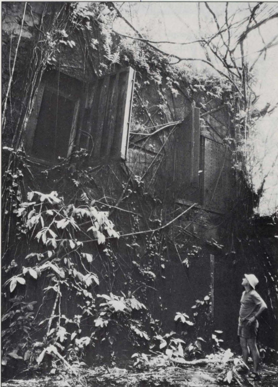
Dick Dewey stands before a bombed-out Japanese headquarters building on Peleliu island.
