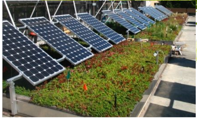
Green roof found on RSTC building on PSU campus
