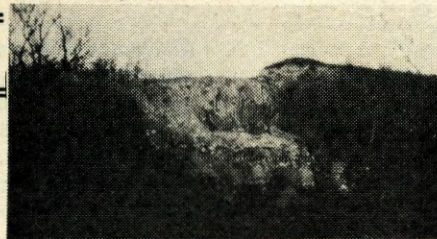
Two views of spoil pushed over the outslope
