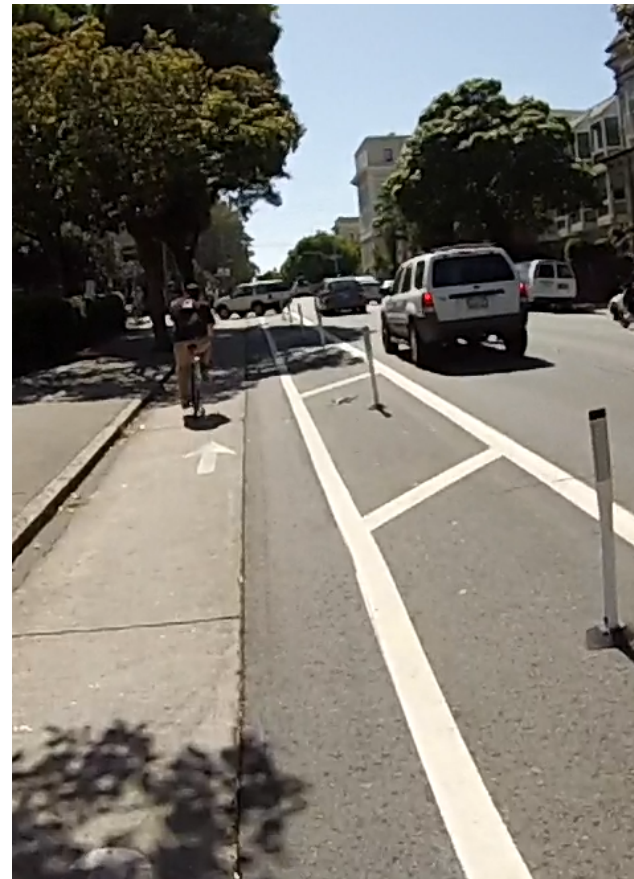
Flexposts and painted buffer (Fell Street, San Francisco)
