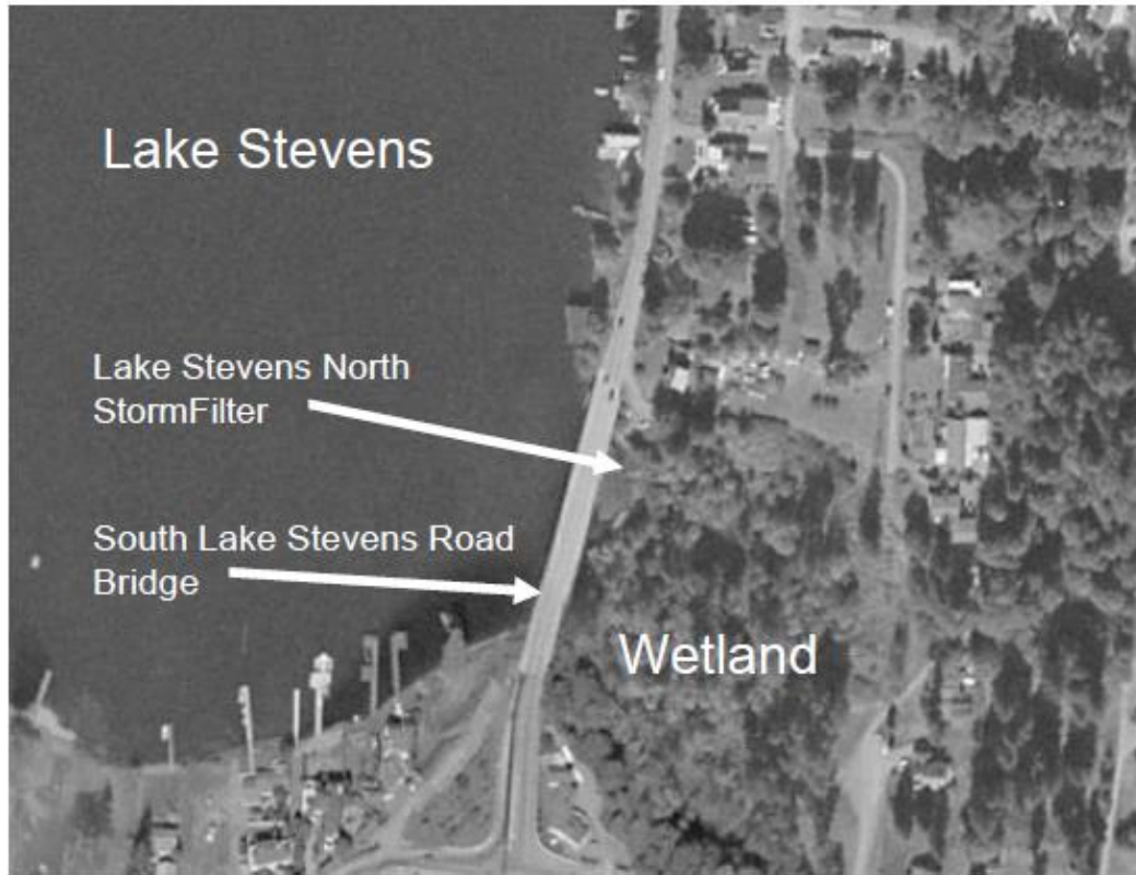
Figure 11: Aerial view of the Lake Stevens North StormFilter site (CONTECH product evaluation, 2006).
