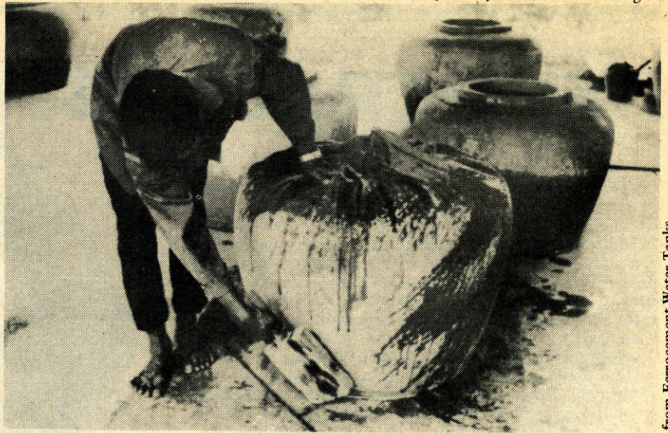
from Ferrocement Water Tanks
