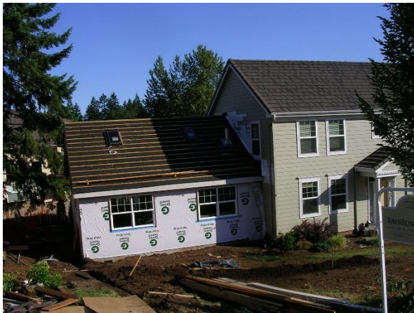
Attached ADU under construction
