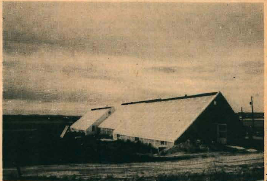
The largest community solar greenhouse (6000 sq. ft.) in the country is located in Cheyenne, Wyoming. Using 312 55-gallon drums for thermal storage, temperatures have not dipped below 40°F in this totally passive solar heated structure. The greenhouse contains an office, storage, bathroom and methane digester which produces heat and sludge. Community citizens actively participated in the design, construction and operation.
