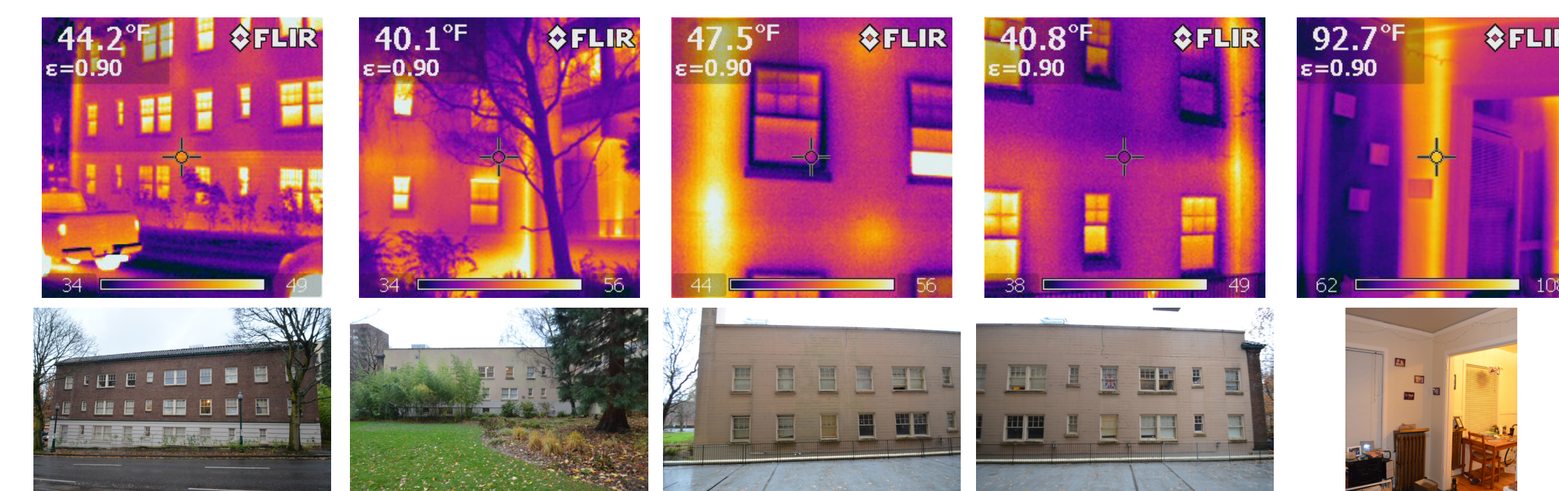
North Facade West Facade South Facade 1 South Facade 2 Interior
