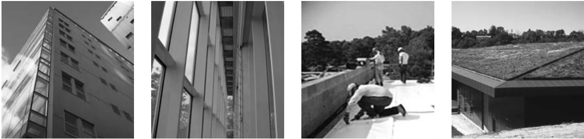
FIGURE 2. Example envelope technologies (from L–R: double skin façade exterior, double skin façade interior 5 , cool roof, green roof 6 ).
