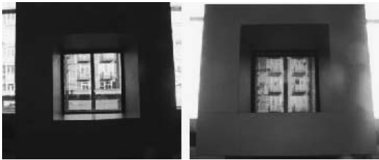
FIGURE 3. Dynamic optical windows are clear (left image) in moderate outside temperatures and translucent (right image) in higher outside temperatures (See http://www.ravenbrick.com/ ).
