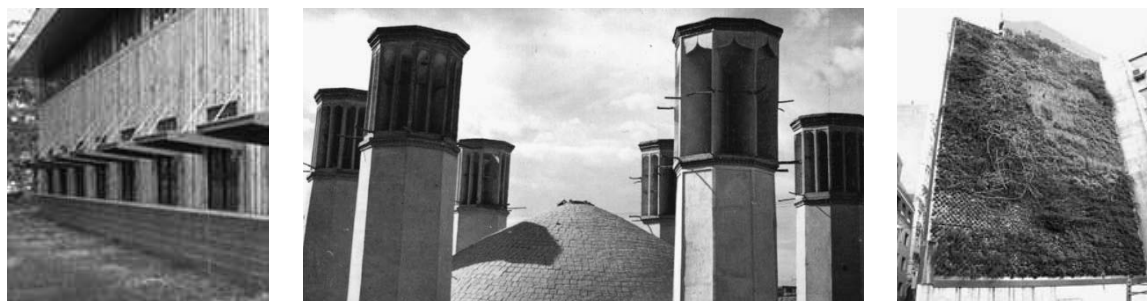
FIGURE 4. Example passive conditioning strategies (from L–R: light shelves that block glare and reflect light deep into interior spaces 8 , wind towers 9 that enable natural ventilation, and a green wall 10 that improves air quality).
