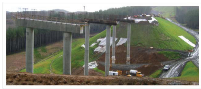
Figure 3.9: Construction of a bridge on the U.S. 20 Pioneer Mountain to Eddyville realignment project. The white tarps on the hillside cover the superficial slope failures, which have resulted in substantial cost and time delays to the project.
