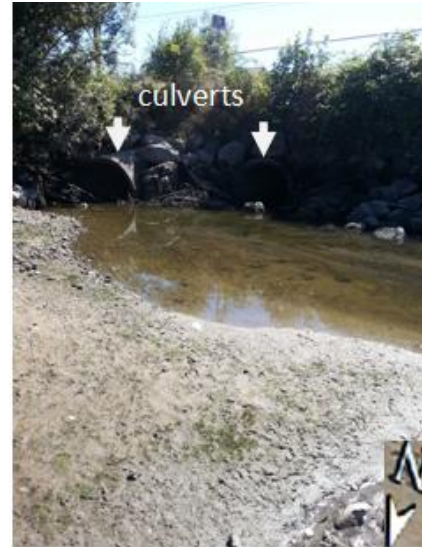
Figure 7: Sediment has built up over 70 years as Clear Creek drops fines during its approach to the northern side of the Bucklin Hill Bridge culverts. September 2014
