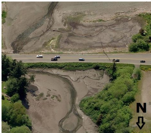
Figure 8: Existing Bucklin Bridge consists of two lanes over an embankment and two 72 inch culverts (Courtesy of Google Earth May 2014)
