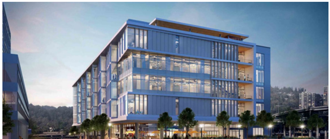
Figure 1: Knight Cancer Institute Research Building Delivered, Third Quarter 2018
