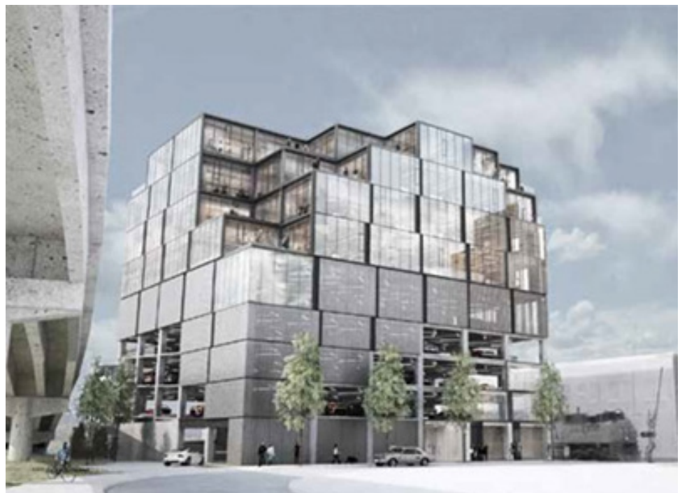
Figure 3: 7 SE Stark Street – Office Space Under Construction – Lloyd District
