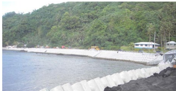
Fig. 21. Erosion control structures such as this seawall in American Samoa can effectively protect coastal infrastructure and development, but are expensive to maintain, and often lead to the conversion of the existing coastal ecosystem into deepwater habitat (photo by E. Gilman).
