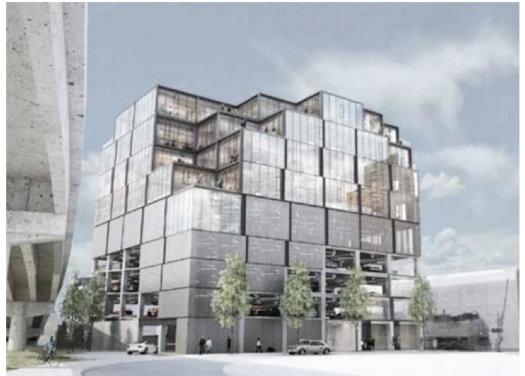
Image 4: 7 SE Stark Street – Under Construction
