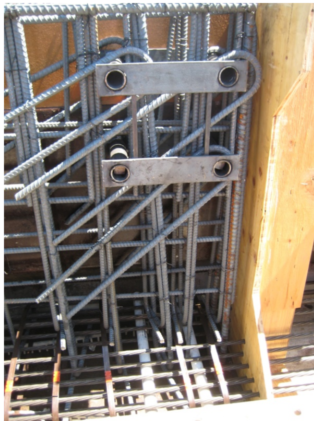
Figure G- 2: Reinforcing Modifications to Test Specimens
