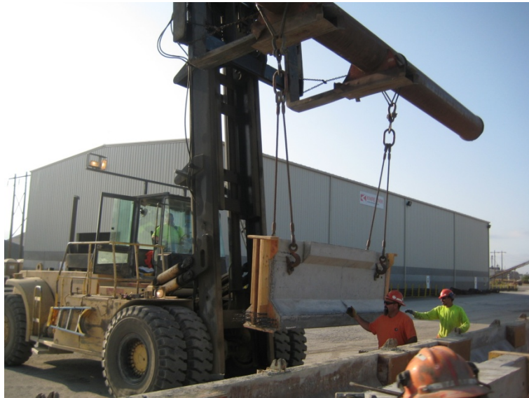
Figure G- 8: Removal of Specimen from Formwork
