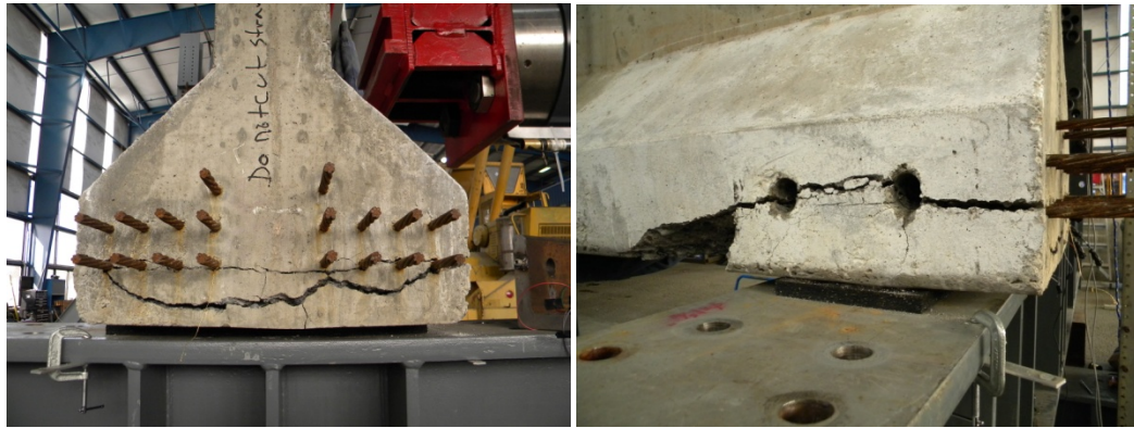
Figure 23: Failure cracks in specimen TB-1.
