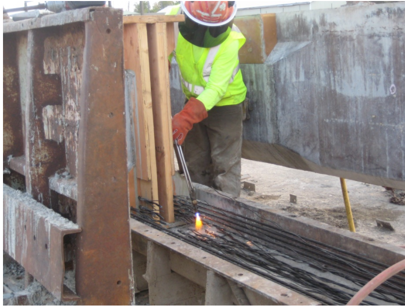
Figure G- 7: Torch Cutting of Prestressing Strand
