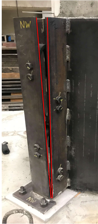
Figure 5.11: Residual hold-down deformation
