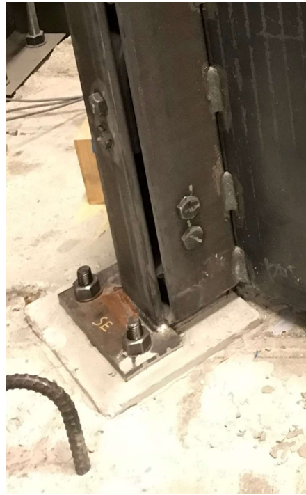
Figure 5.5: Hold-down base plate
