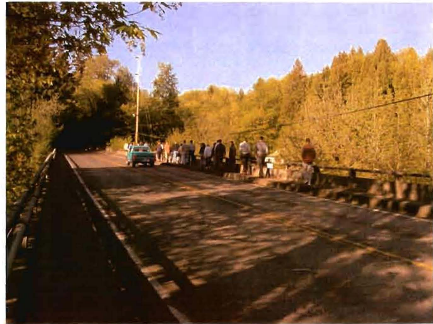
Bridge Over Tualatin River, Stafford Road
