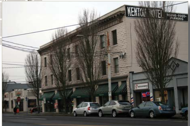
The Masonic Lodge (left) and the Kenton Hotel Building (above) are located on Denver Avenue. The Paul Bunyan statue (Denver Avenue and Interstate), a signature of the neighborhood, was erected for the Oregon centennial exposition in 1959.
