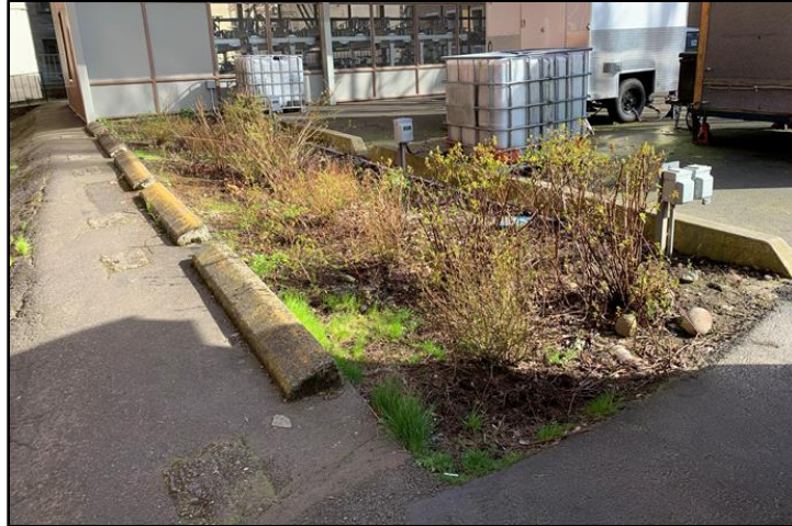
Figure 7. Bioswale on Library Bicycle Garage (2021).
