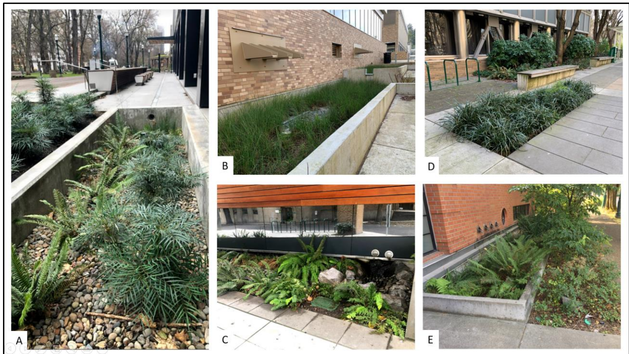
Figure 4. Flow-Through Planters on Campus. A: FMH, B: Peter Stott, C: KMC, D: Cramer Hall, and E: Helen Gordon (2020-2021).
