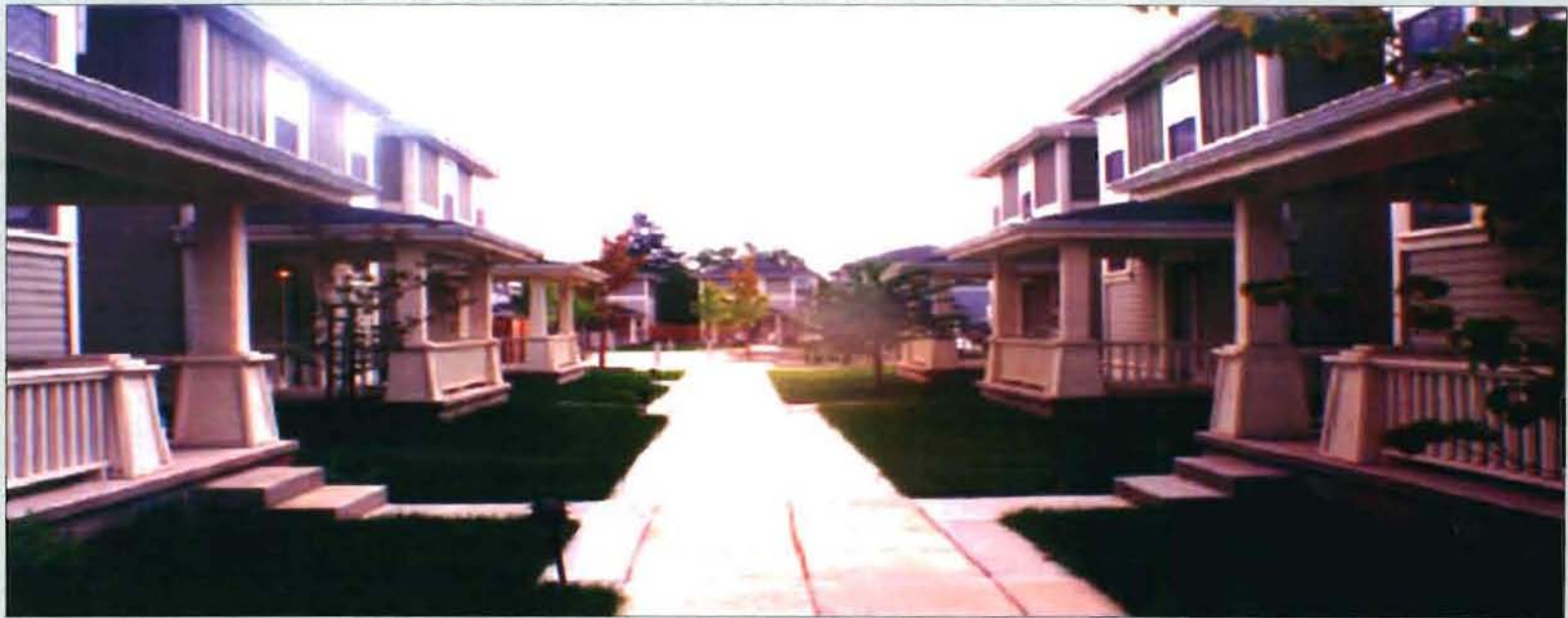
Central walk at Bungalow Court Condominiums, Portland, Oregon.
