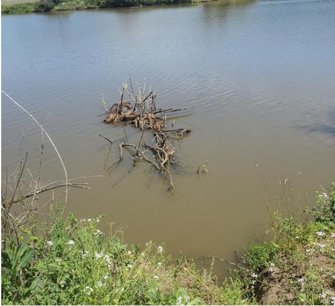
Figure 2: Small Woody debris structure installation (Photo credit: J. Holley, 2020).
