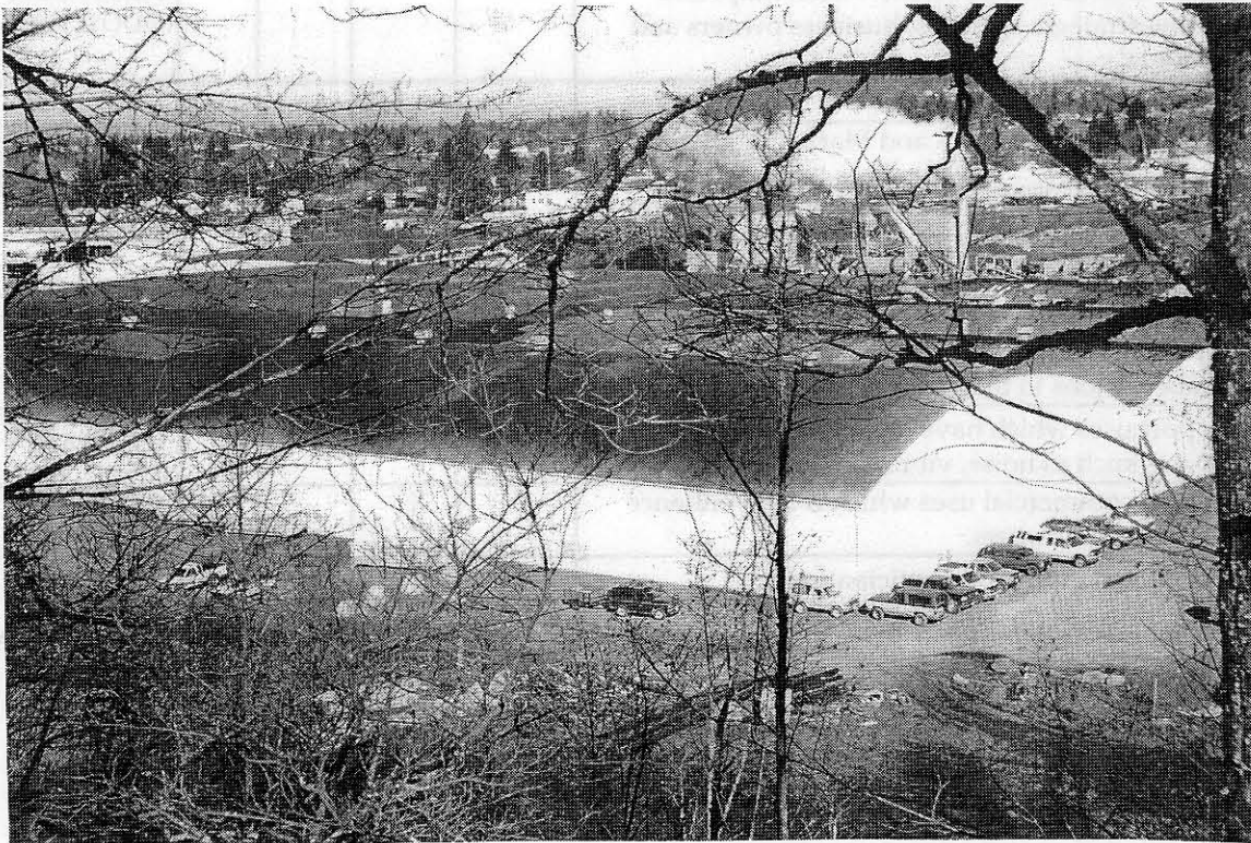
The Freeway Land Company site east of I-205 and south of Foster Road is the largest industrial site in Outer Southeast.
